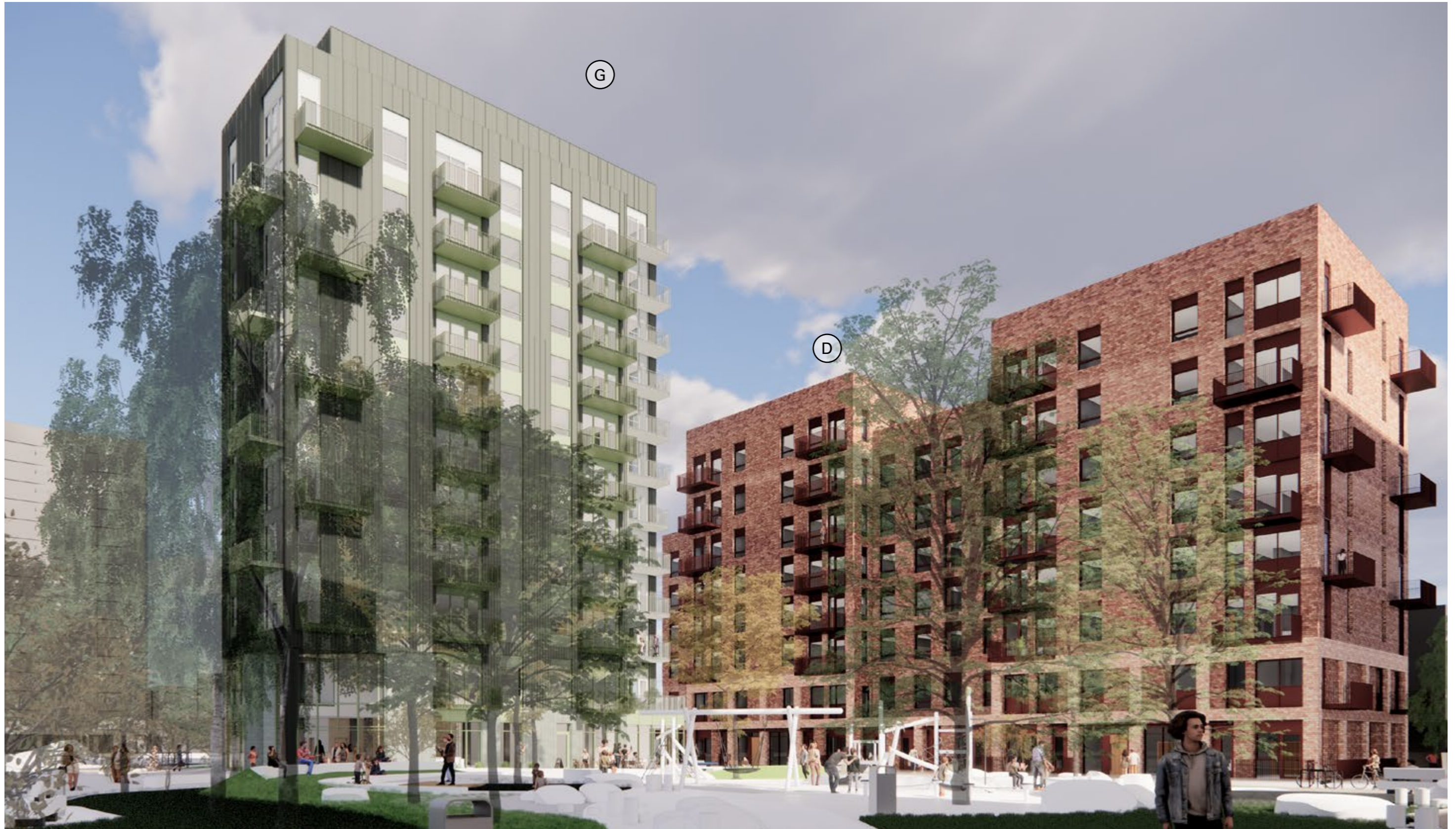
View looking southeast from Plot B
